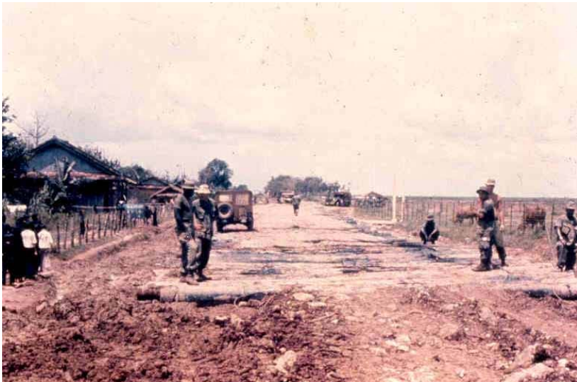
Military Service Road (MSR) Zinc – placing corduroy road, 34 th Engineer Battalion, September 1969. A “corduroy road” is an ancient technique of using tree trunks lined up side by side to provide support on muddy soil.
